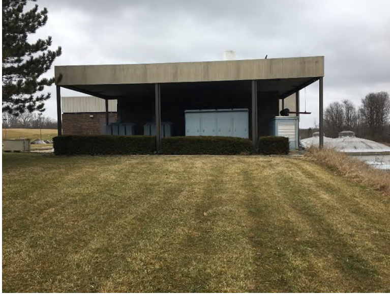
Picture 15: Facing north, south of Primary Clarifier Building, transformer yard
