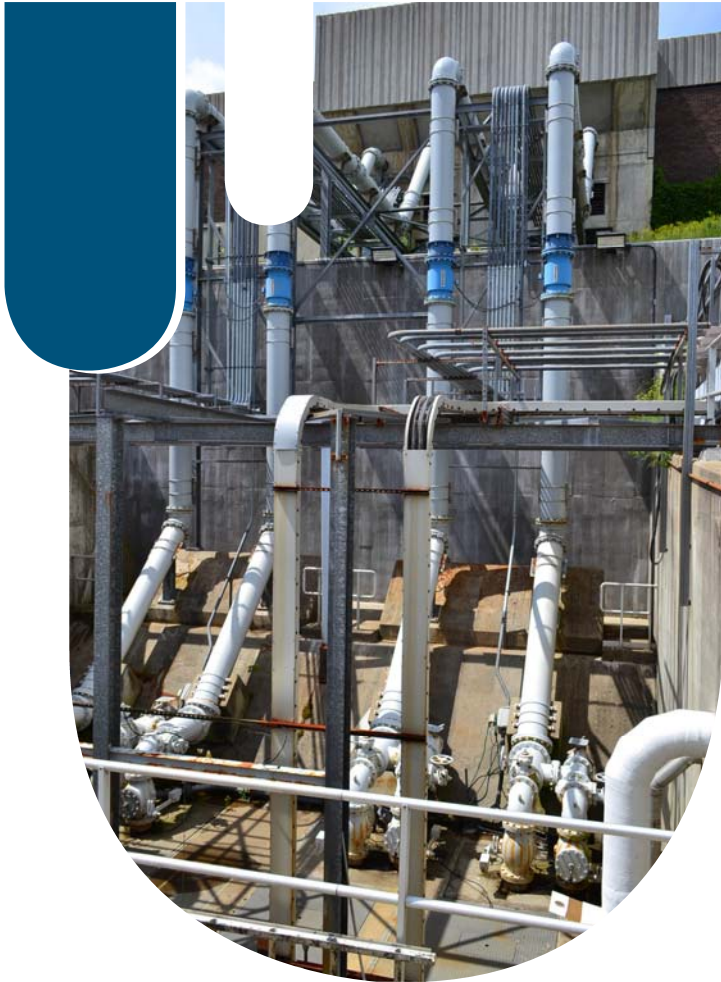
WWTP Major Capital Improvements
