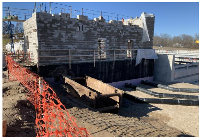
Photo 6: Blower Building CMU Installation
