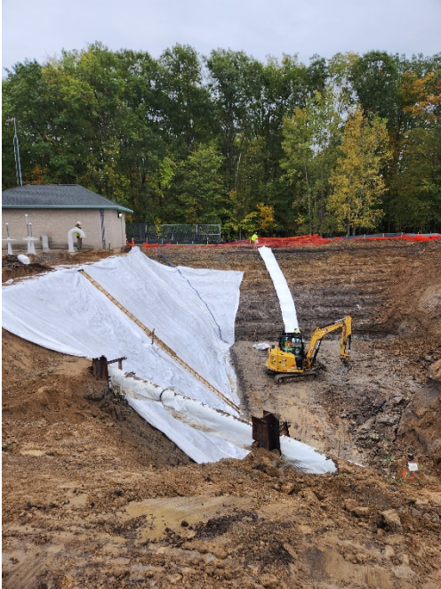
Photo 1: Protection of slope and perimeter drain placement during EQ basin excavation.
