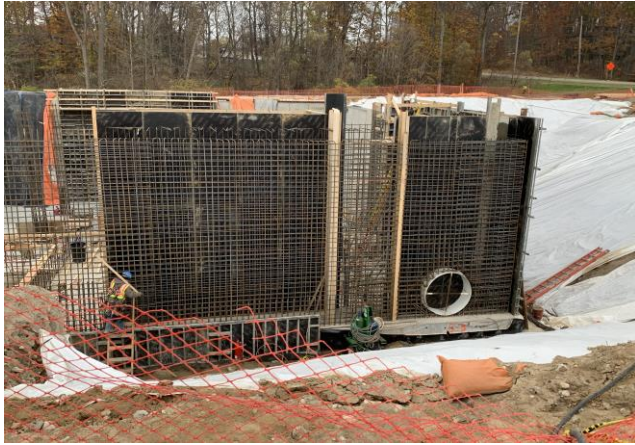
Photo 7: Headworks Building Wall Resteel
