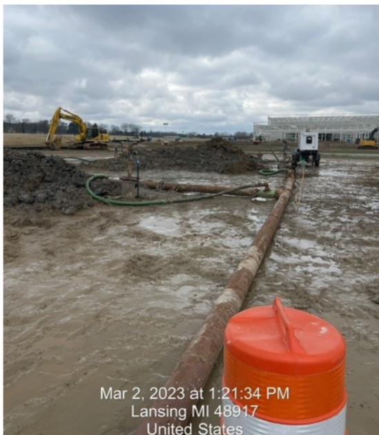
Photo #1 – Discharge Pipe
