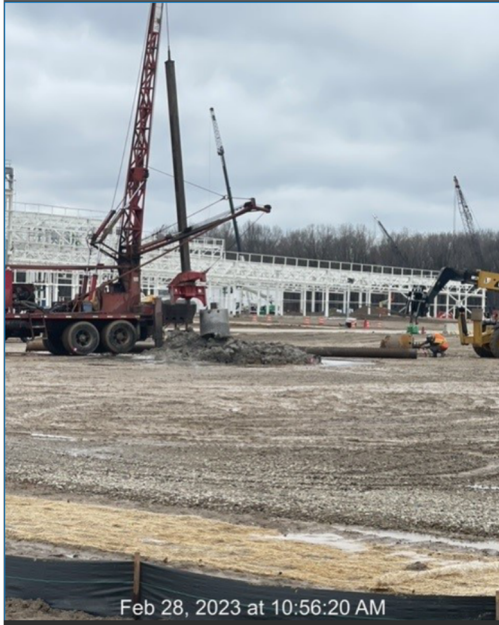
Photo #2 – Well Drilling Rig
