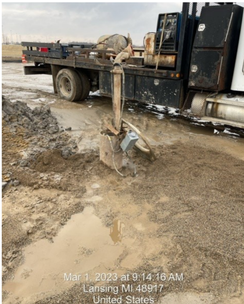
Photo #3 – Deep Well Casing
