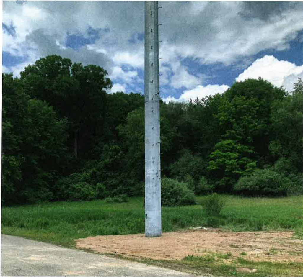
Figure 1. Recently Installed Pole at East Lansing WWRF
