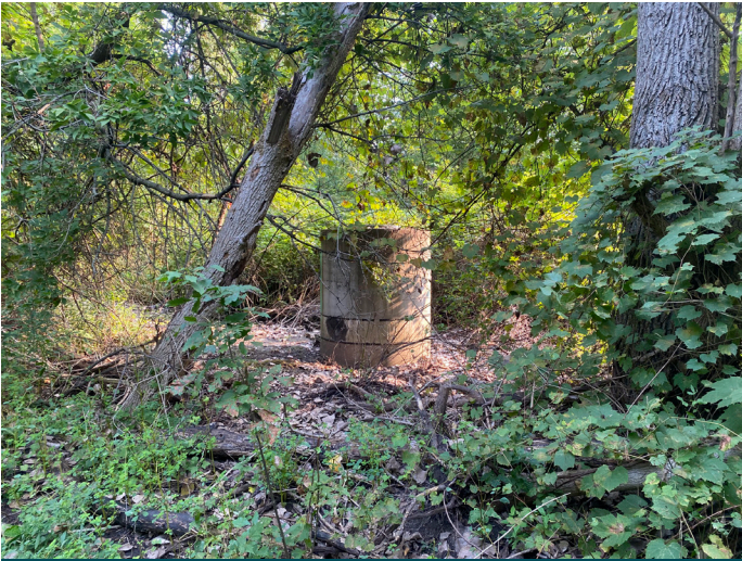
Manholes will be extended beyond the base flood elevation with sealed and joined sections.
